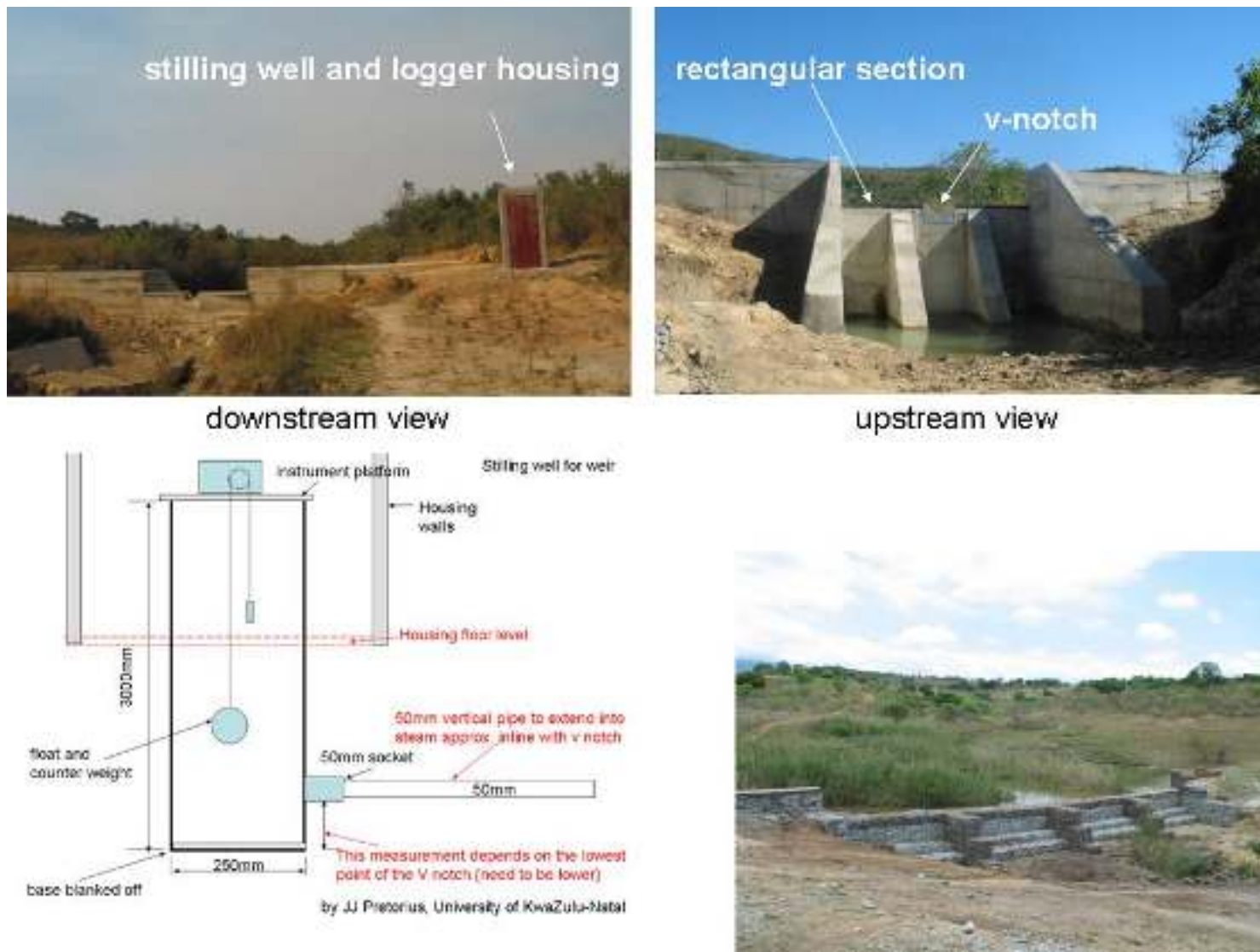
Figure 3.5: Installed buttress weir (top left, top right) with design and location of stilling well (bottom left), gabion dam (bottom right)
